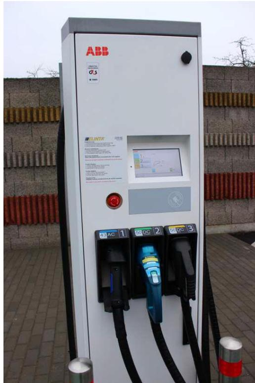
**Figure 5.** ABB concern fast charging station (It stands in Vevis at A2 highway). Apparently, the station provides charging both AC in MODE 3 and DC in MODE 4 by both standarts)
